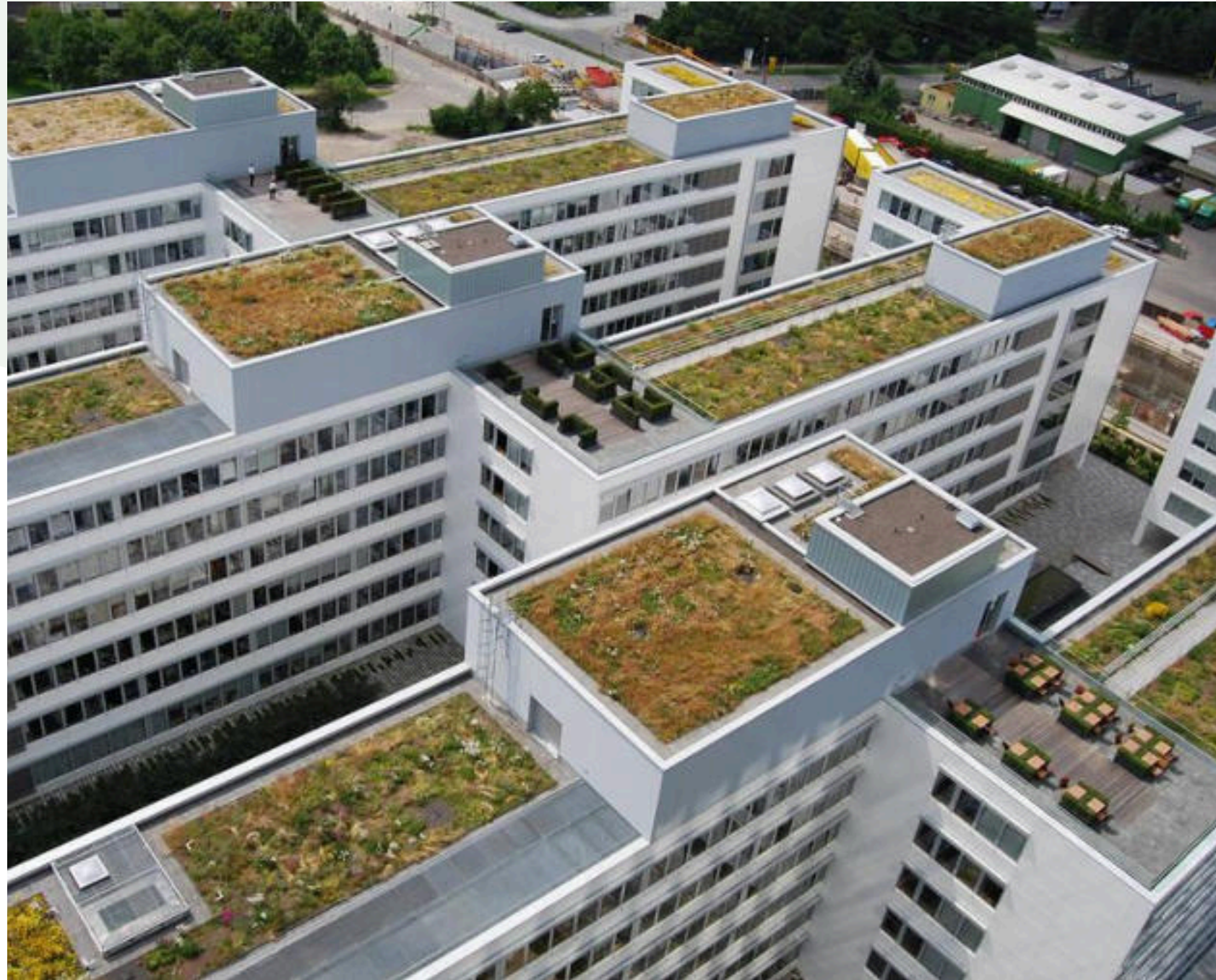
© Optigrün international AG, 2026 The Green Roofs at the EnBW Administrative Complex
